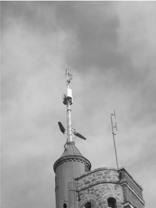
**Fig. 31.19.** Practical example of a translator or gap-filler site; the 2 (log periodic) receiving antennas are located in the lower part of the extended pinnacle of the tower, the 3 transmitting antennas (8-element bays) are located in its upper part
