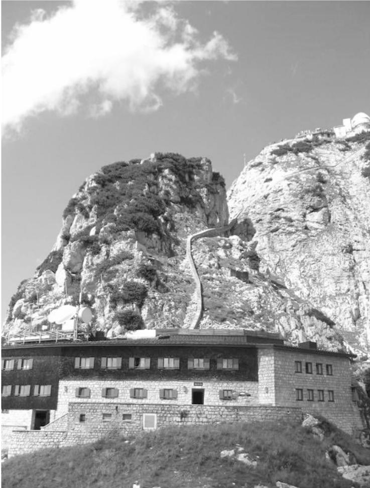
**Fig. 46.3.** Transmission station Wendelstein, Bayerischer Rundfunk, directional radio antennas and cable duct for the transmission cable clearly recognizable
