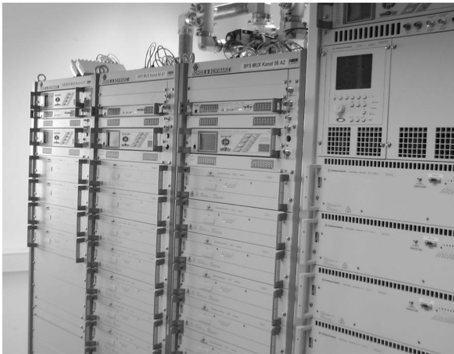
**Fig. 46.5.** DVB-T transmitter racks, transmitter station Wendelstein, Bayerischer Rundfunk
